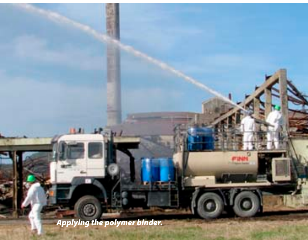
Polymer binding ash and dust into a spongy blanket about 20 mm deep.
